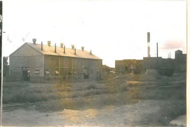
Cleveland Quarries Co. Blacksmith Shop South Amherst
