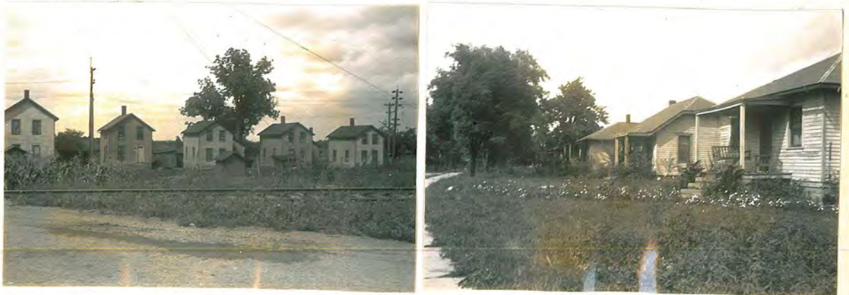
Quarry Houses at South Amherst
