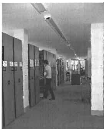
Completed compact shelving
